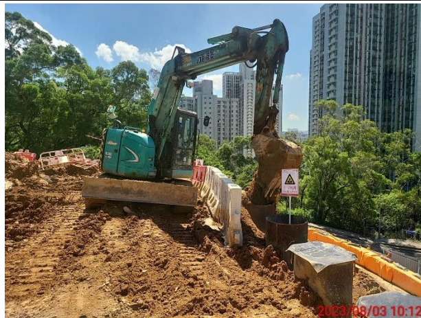
Construction activities: Backfill
