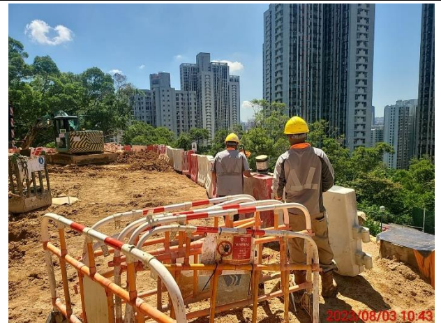
Construction activities: Setup water-barrier and housekeeping
